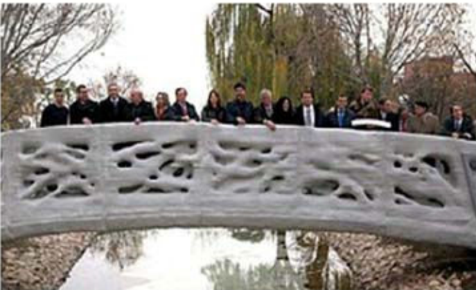
3D printed bridge with the D-Shape technology. The first structure of this type in the world
